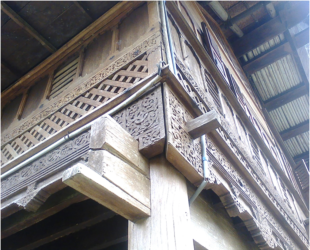
Figure 7 Arabic Calligraphy is a motif carved in the middle of the wall of Tgk Chiek Awe Geutah Rumah Aceh.
